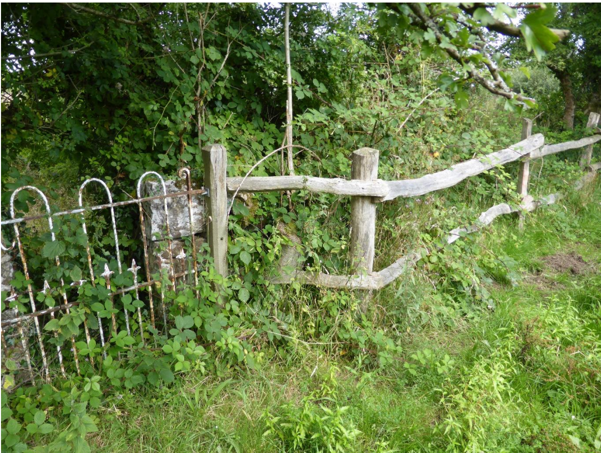
Our own cleft post and rail fence, using oak from a woodland manager near Llandeilo
